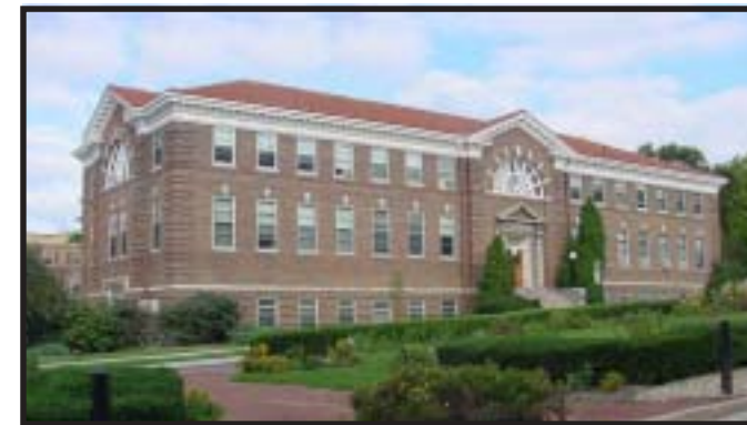
Agricultural Engineering Building at 460 Henry Mall.
